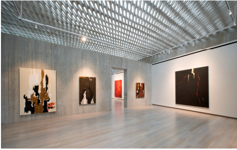
Installation view of the inaugural exhibition. The experience of the collection is enlivened by natural light that enters the galleries through a series of skylights over a cast-in-place, perforated concrete ceiling.
