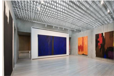
Installation view of the inaugural exhibition. The experience of the collection is enlivened by natural light that enters the galleries through a series of skylights over a cast-in-place, perforated concrete ceiling.
